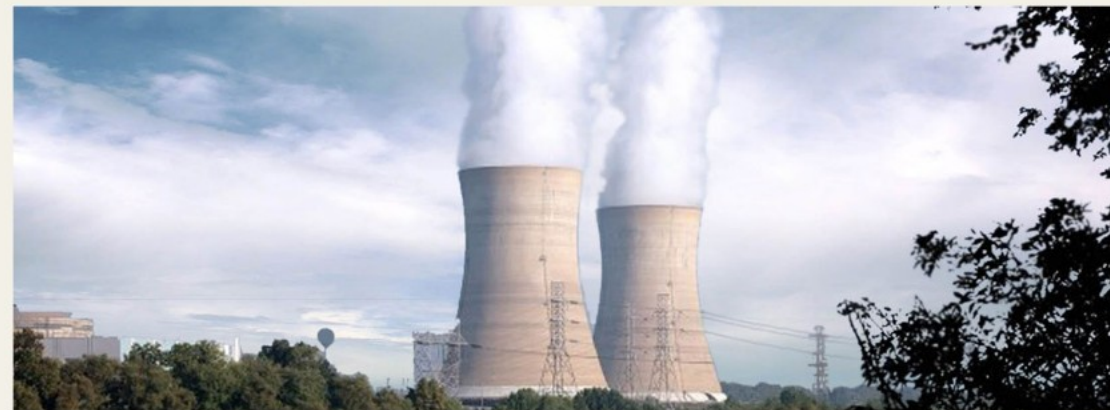
Crane Clean Energy Center · 既存施設写真：Constellation
